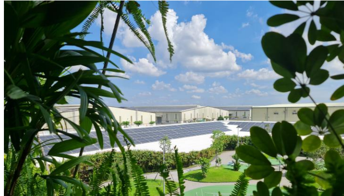
Figure 17: Rooftop solar installation at Jacob Factory, Binh Duong, Vietnam (©dena / Stefan Schirmer)
